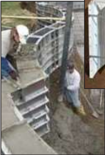
Concrete Floor Casting
