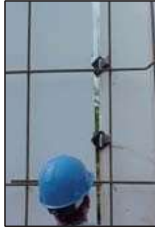
The next piece of insulation is placed using the recesses created to accommodate the plates with the fasteners and spacers.
