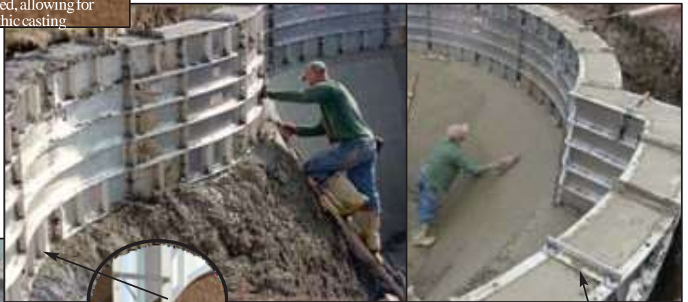
Pool Floor Finishing Process in Transition with Walls
