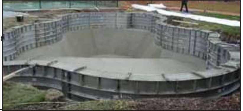
"Mountain Lake" pool of 26' x 52' with monolithic casting
