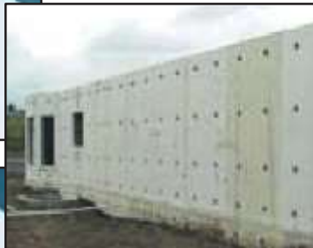
Once the concrete pouring and stripping work is completed, the G, I, and T profiles are used to receive the application of exterior finishes.
