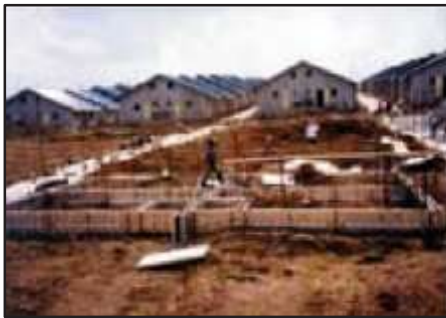
Quadruplex Housing Project, Philippines
