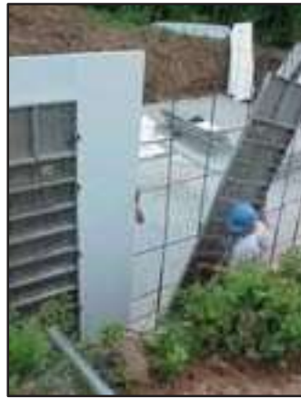
The placement process continues on all walls and adjustments are made with the "I" profiles on the "T" walls. When the panel placement is finished, the pouring process begins.
