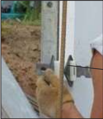
The WTF insulation board and plate fastener are designed to fit perfectly into the holes.
