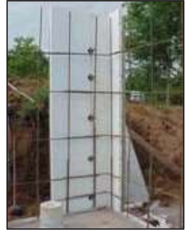
The next piece of insulation is placed using the recesses created to accommodate the plates with the fasteners and spacers.
