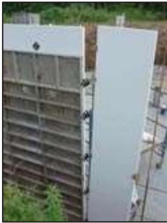
The placement process continues on all walls and adjustments are made with the "I" profiles on the "T" walls. When the panel placement is finished, the pouring process begins.
