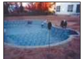
Installation of vinyl sheeting in a 26' x 52' "Mountain Lake" pool
