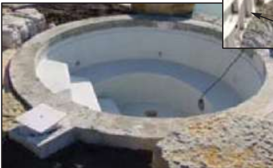
6-foot diameter spa under construction
